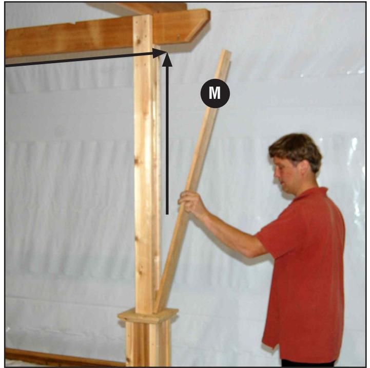
10. Attach Post Trim to post with eight 1 1/2" Finish Nails (FF) in positions shown.
