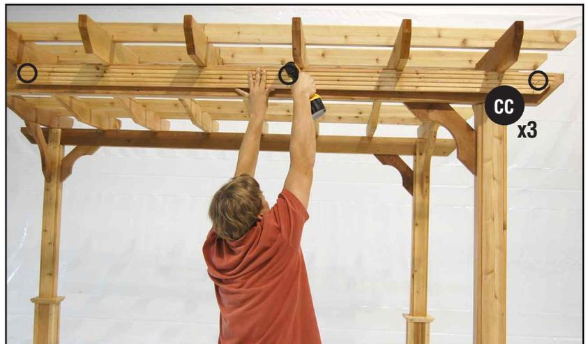
3. Locate one Short Beam Trim (S). Place Short Beam Trim snug against end of Long Beam Trim and snug against rafters. Attach using two 2 1/2" Screws (CC) at each end of trim.
