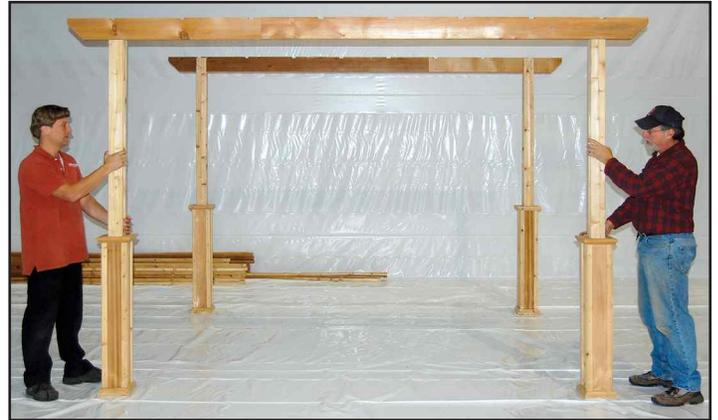
5. Line up the notches on one rafter assembly with the notches on the far end of each post and beam assembly. Push down on rafter to seat.
