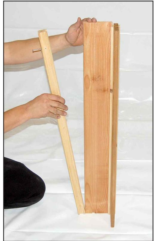
**NOTE: The A and B sides will protrude on one end. This will be the ground end of the post base assembly.**
