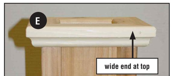
13. Attach top trim using four 2" Finish Nails (EE) installed over the side boards at the center of each side.
